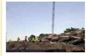
Going, going, gone! Schine Hall's final demolition in August.
